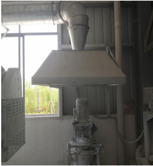
颜料搅拌废气集气罩
